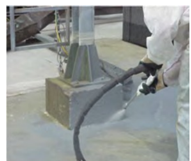
Application of MasterSeal M 689
