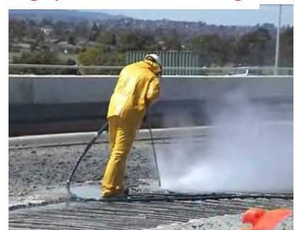
Mechanical preparation for the substrate, Blast Cleaning
